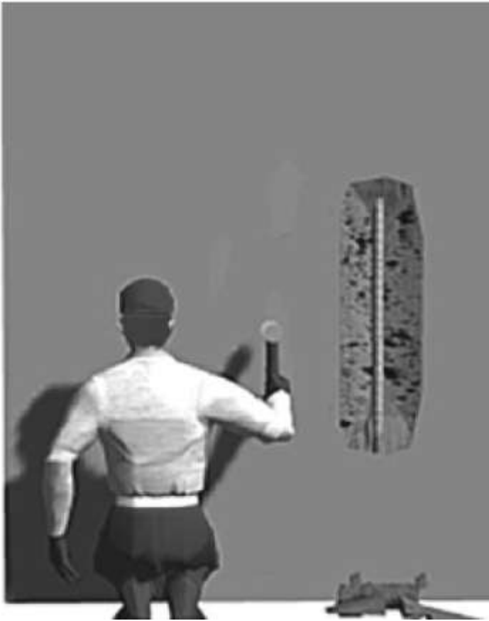
Removal of loose concrete
